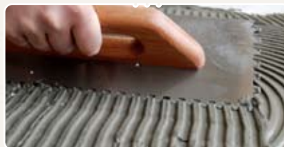
Thinset mortar application
