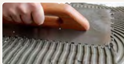
application de ciment-colle
