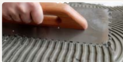
application de ciment-colle
