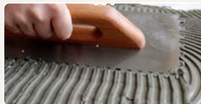
Application de ciment-colle
