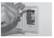
5. Route wires coming from the wall through the hole of the mounting base and make the required connections using the "Four-wire installation" figure, and using the supplied solderless connectors. A pair of wires (black) must be connected to the power source (120-208-240 VAC) and another pair (yellow) must be connected to the heating cable (refer to the drawings displayed on the back of the
