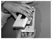
4. Align and secure the mounting base to the connection box using the two screws supplied;
