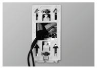
7. Align the little slots located on the top of the thermostat with those on the the mounting base and secure the thermostat to the mounting base. Note that you can also position the thermostat on the left or the right side of the junction box (see the illustrations below). Then, tighten the screw at the bottom of the unit.
