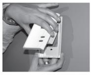
4. Align and secure the mounting base to the connection box using the two screws supplied.
